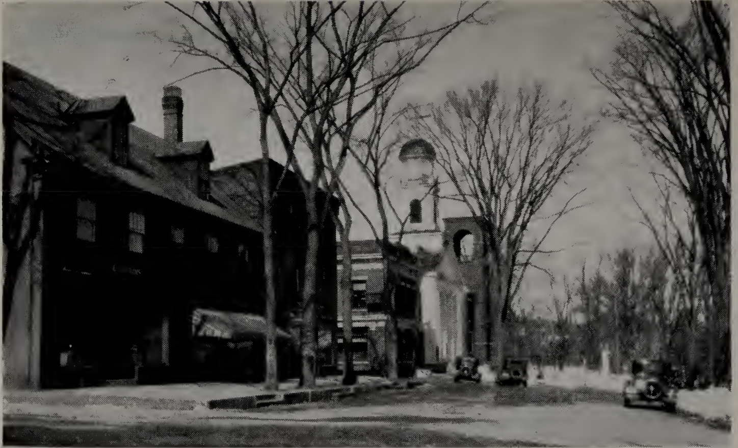
The Old Brick, Moor Russell's Store, 1822, at the corner of Highland and Main Streets, razed for the site of the post office in 1936.
